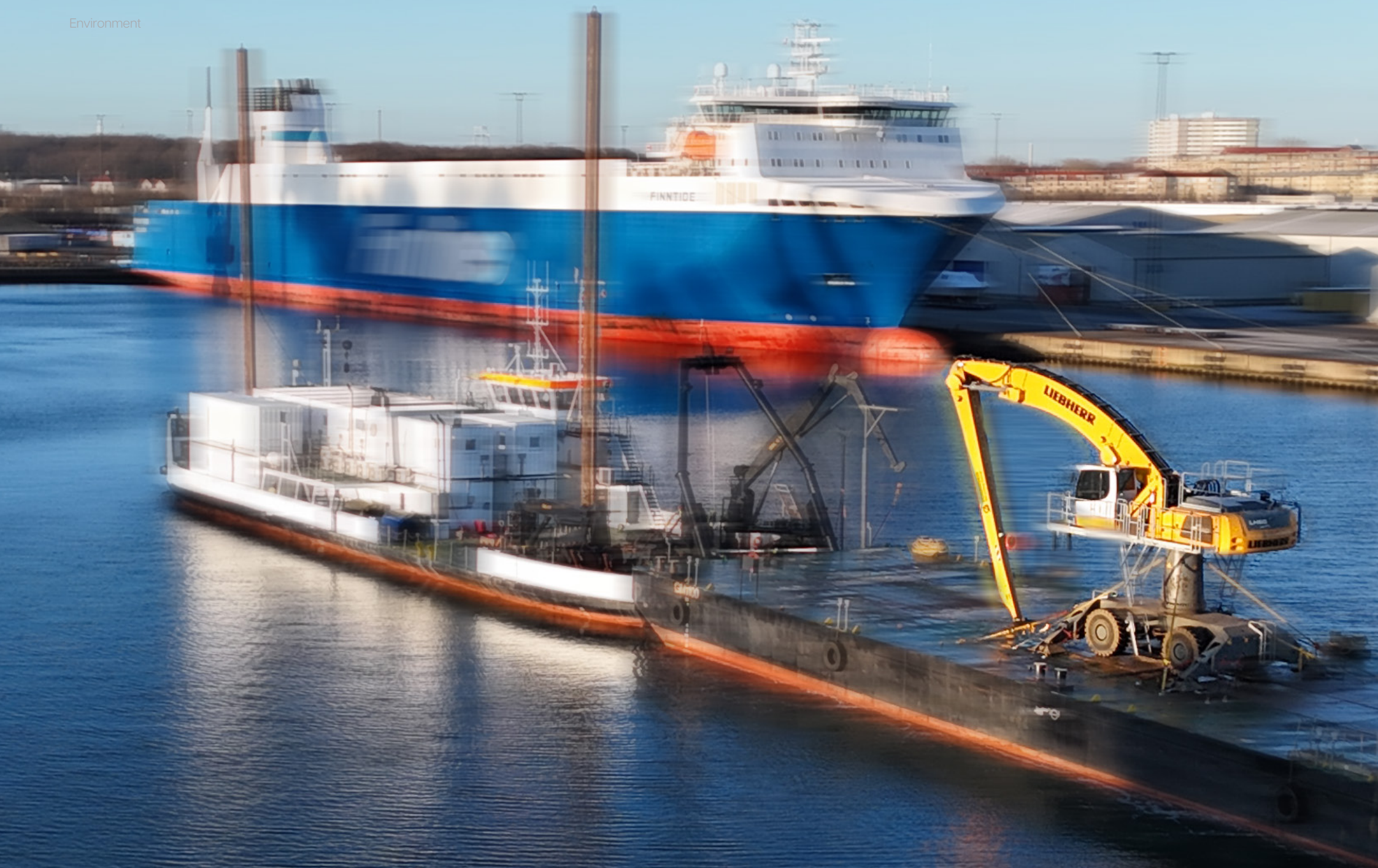
Image: Relocation of a Liebherr crane from the site in Kolding to the site in Aarhus via barge.
